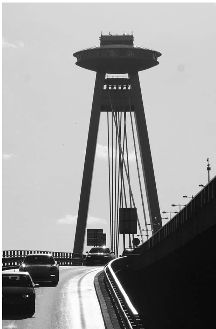
Most (Bridge) SNP - UFO Tower
